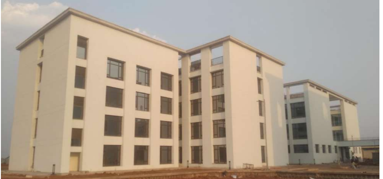
Outside view of MDC Block
